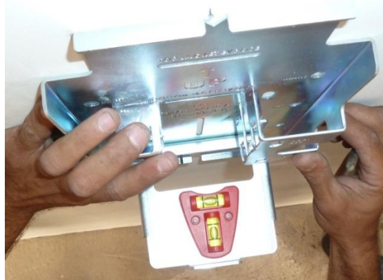
Figure 64: Leveling Plate is Level
