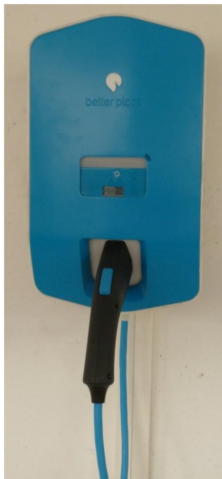
Figure 86: Installed Single Socket Wall CS
