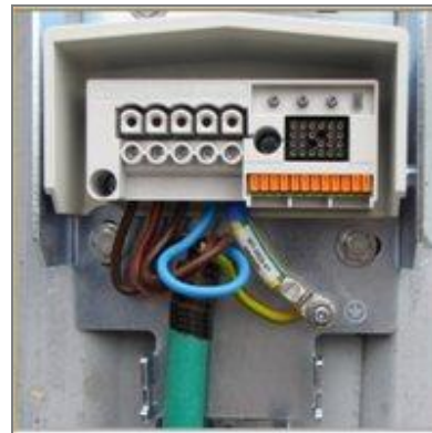
Figure 44: Power and Ground Cables Connected to the Fast Connector
