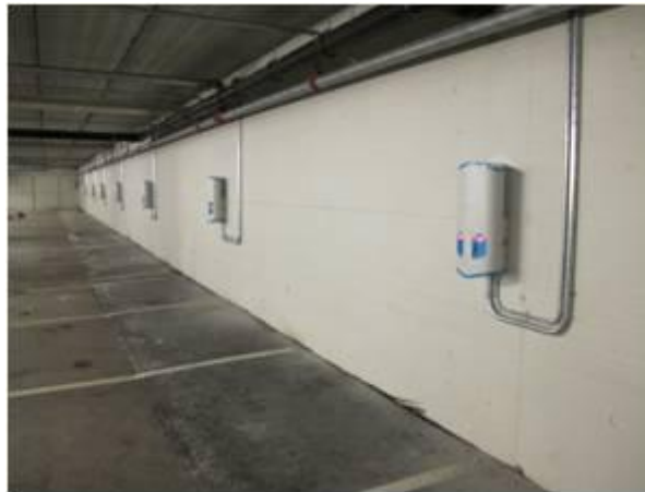
Figure 104: Wall CSs Installed
