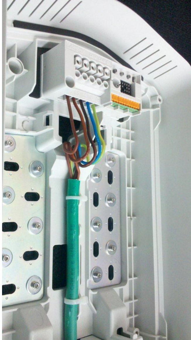
Figure 79: Power Cable Strands in 'S' Configuration
