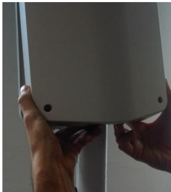
Figure 114: Slide the Top Assembly Infrastructure Adapter on Pole
