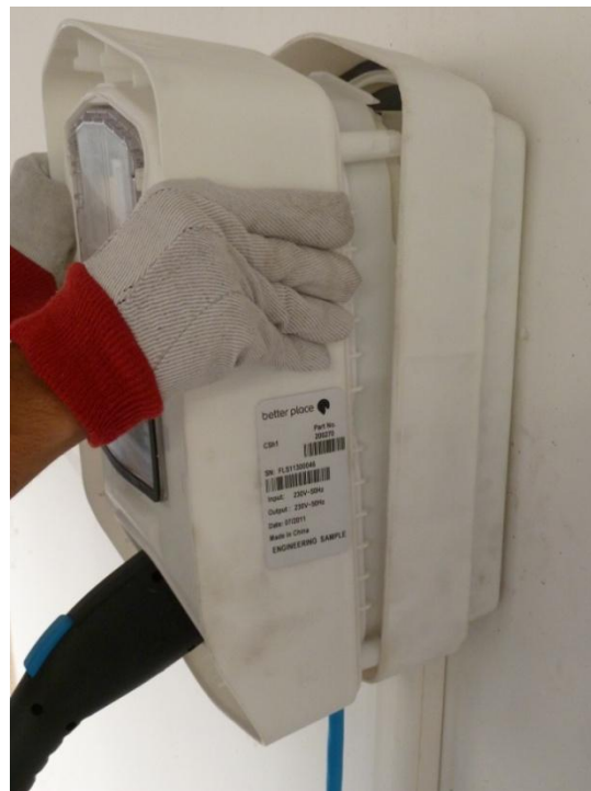
Figure 108: Attach the Wall CS to the Infrastructure Adapter
