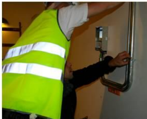
Figure 99: Install the Conduit and Bracket
