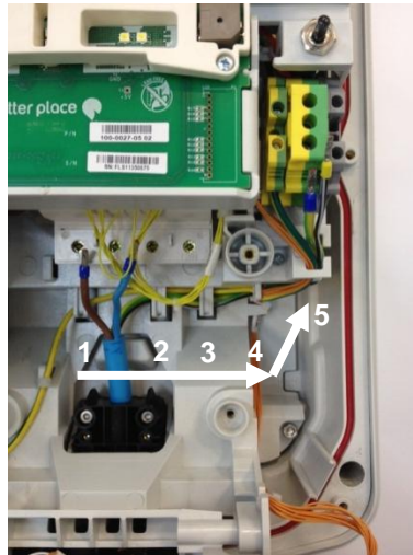
Figure 151: Route Wires through Plastic Borders
