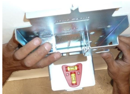
Figure 8: Mark the Wall with Leveling Jig
