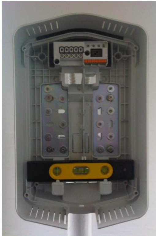
Figure 125: Level the Infrastructure Adapter
