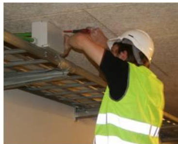
Figure 4: Install Junction Box and Power Raceway
