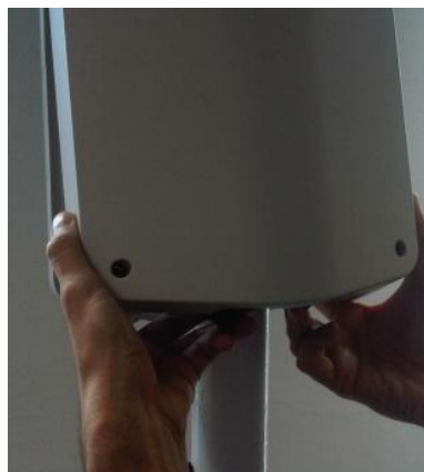
Figure 134: Slide the Top Assembly Infrastructure Adapter on Pole
