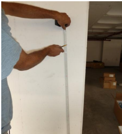
Figure 62: Measure 157 cm for the Single Socket Wall CS
