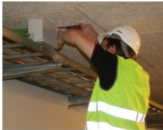
Figure 98: Install the Junction Box and Power Raceway
