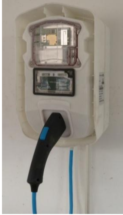
Figure 11: Installed Single Socket Wall CS
