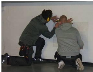
Figure 3: Determine Bracket Location
