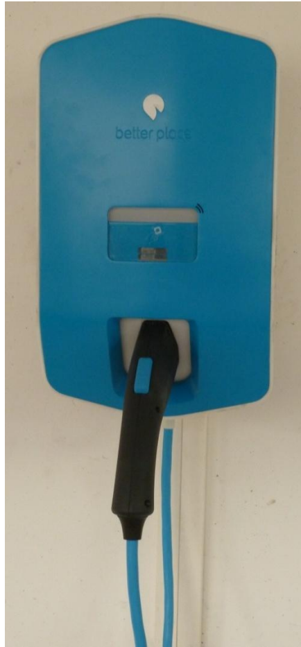
Figure 109: Installed Single Socket Wall CS
