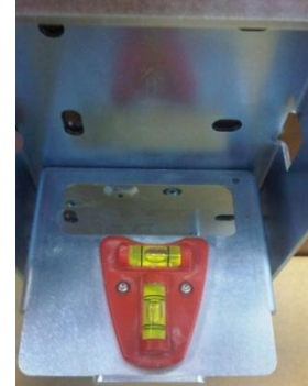
Figure 37: Bracket is Level
