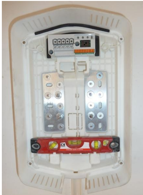
Figure 75: Leveling the Infrastructure Adapter
