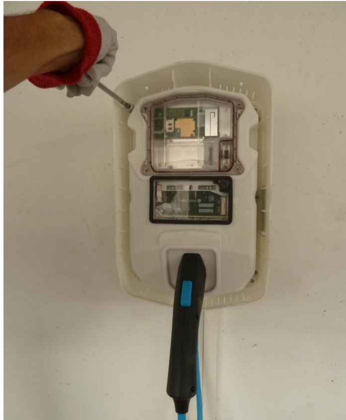
Figure 82: Tighten Single Socket Wall CS Screws
