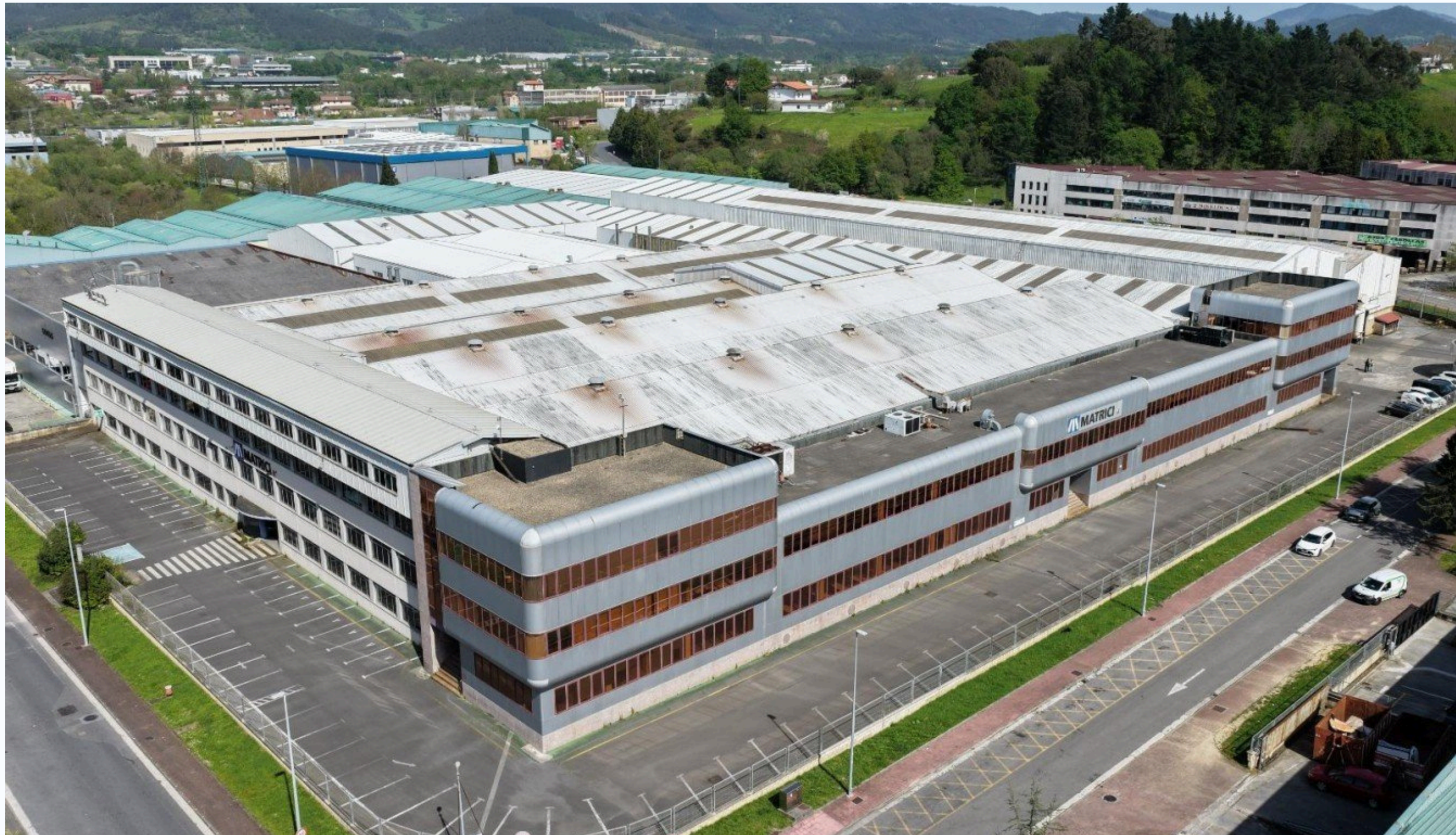
Panoramic aerial view of the warehouse
